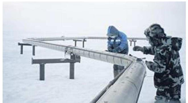
Fig. 8. A heated pipeline with IRHS installed on it.
